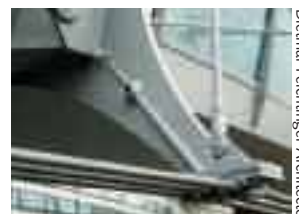
Detail of vertebra with fixation of prestressed circular cables.
