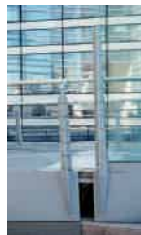
Balustrade with horizontal prestressed cables and inox tube for handrail, vertical posts integrating light.
