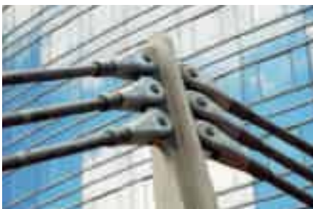
Suspension cables fixed to vertebra.
